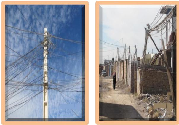
**Figure 3.** Condition of electrical wiring, passages and buildings of the complex (Resource: author 2012)
