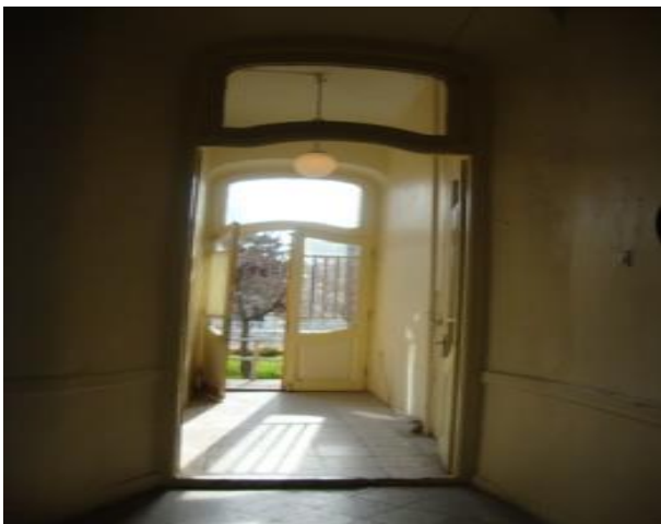
Figure 15. High and Brushed Openings in southern facade
