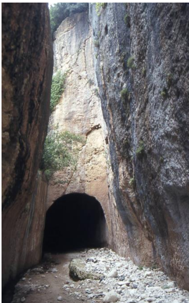
Figure 3. Entrance to the upstream first tunnel, with 5.8 m height and 6.3 m width, in Seleuceia Pieria (photo: Ü. Öziş).
